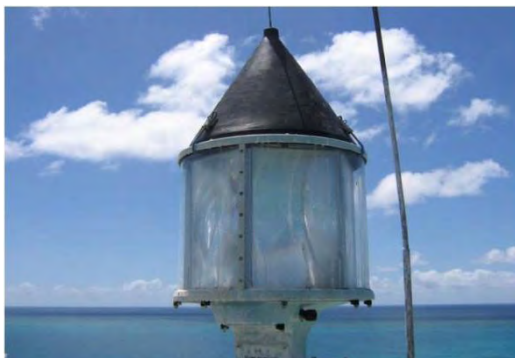
Figure 2. Adding cones to flat lantern surfaces
